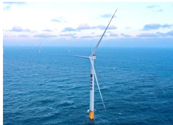
The International Fuyuan West Offshore Wind Farm, with largest installed capacity of the country's highland wind power bases
